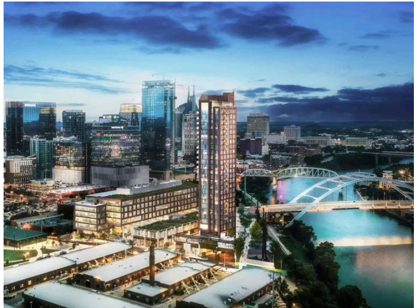
Peabody Union's apartments will provide views of the Cumberland River. Image courtesy of Stiles|Hensler and PGIM Real Estate
